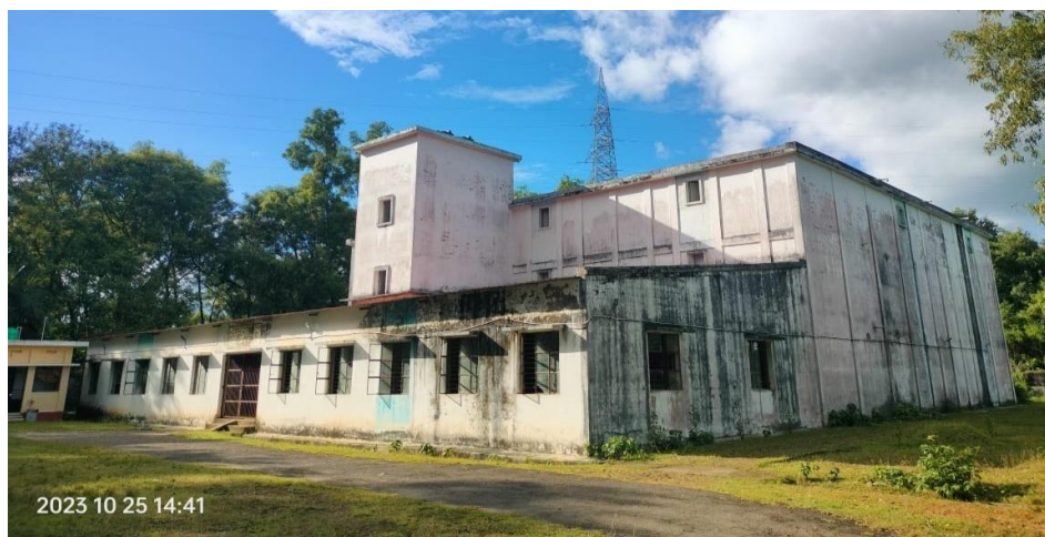
Figure 1: Multipurpose cold storage (South Tripura), Date: 25/10/2023
