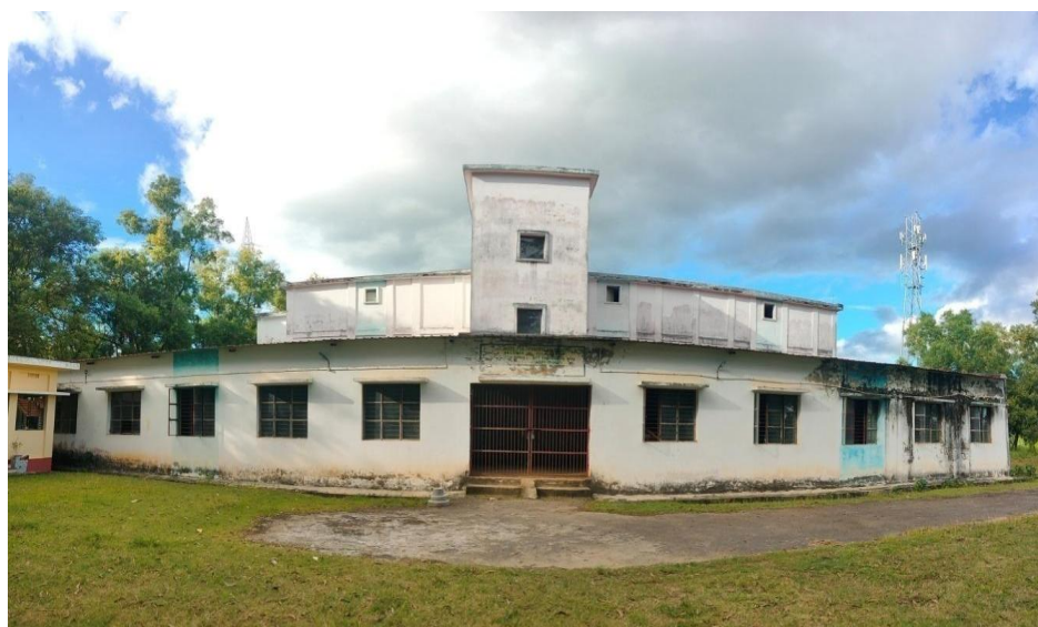
Figure 2: Multipurpose cold storage (South Tripura), Date: 25/10/2023
